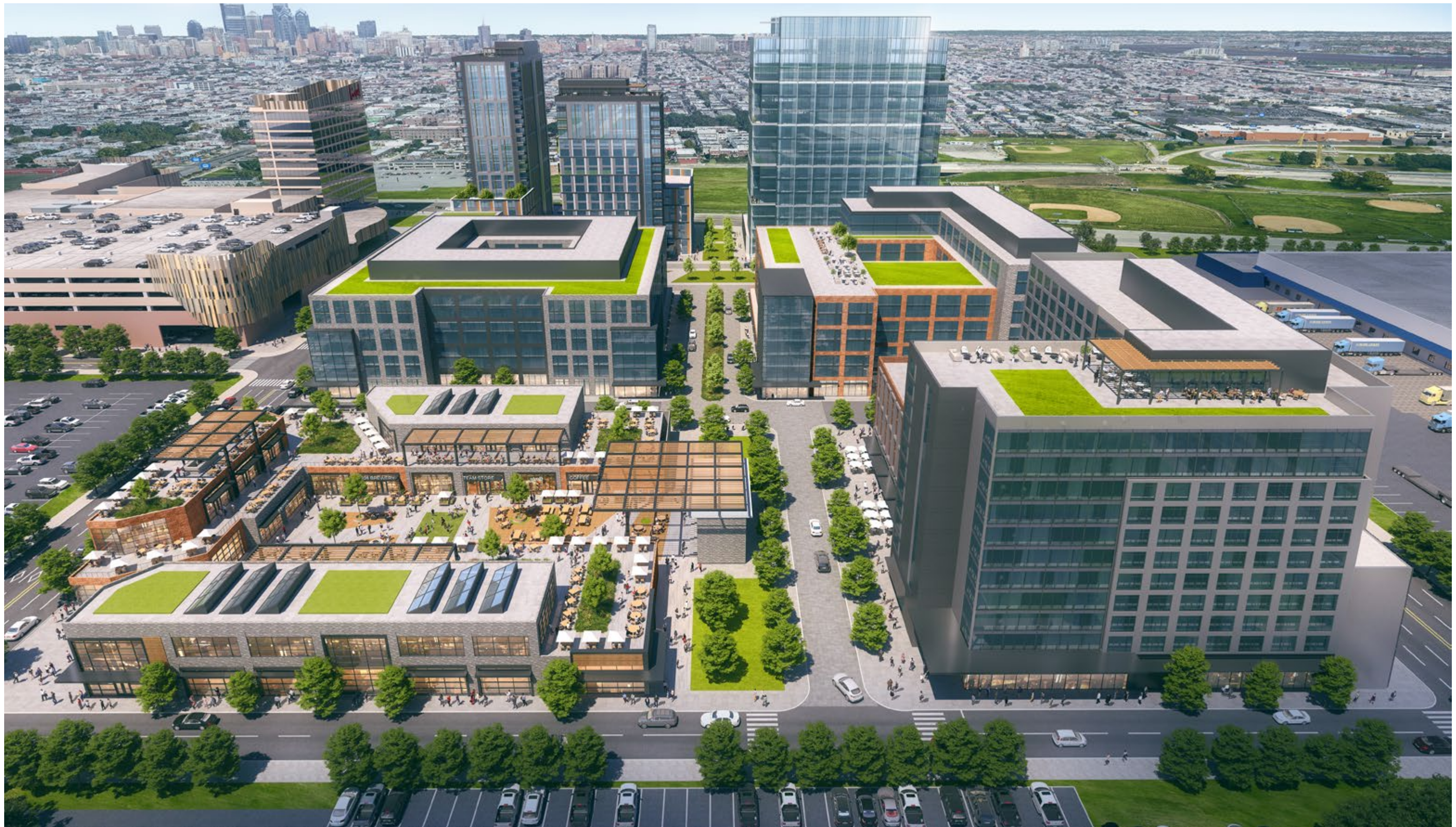
Aerial Looking North
